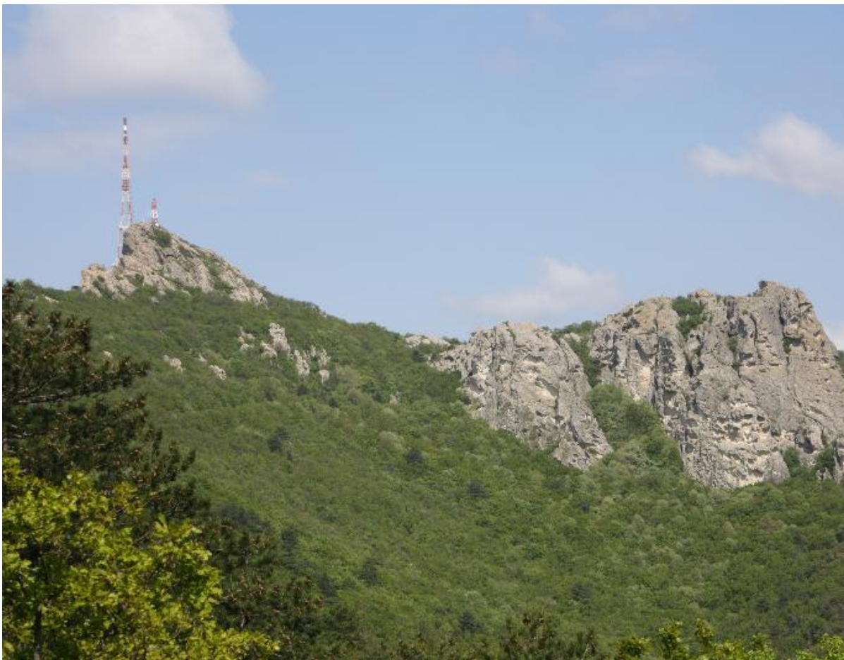
Kapsalo radio mast
